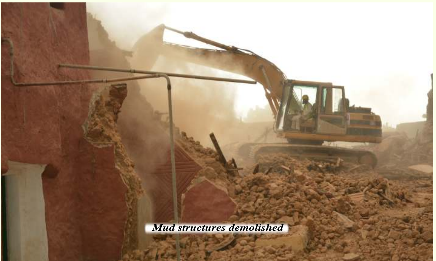
Mud structures demolished
